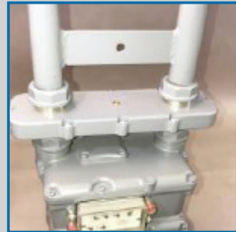
6. Turn back to BY-PASS and remove the meter nut plug
