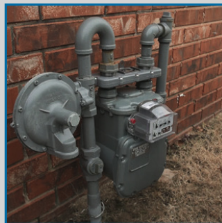
6. Connect the outlet side of the new meter
