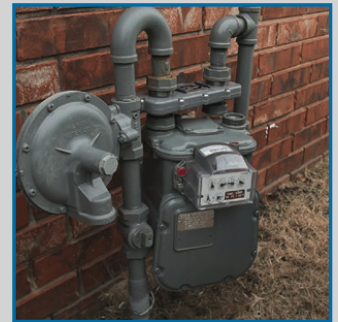
4. Connect the inlet side of the new meter
