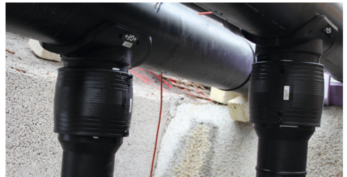
Simple and fast connection: ELGEF Plus branch saddles d450 mm x 225 mm.
