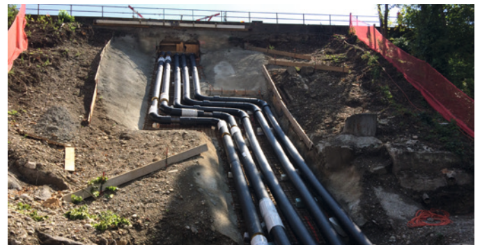
Torfeld Telli section: 2 steel and 3 PE lines.
