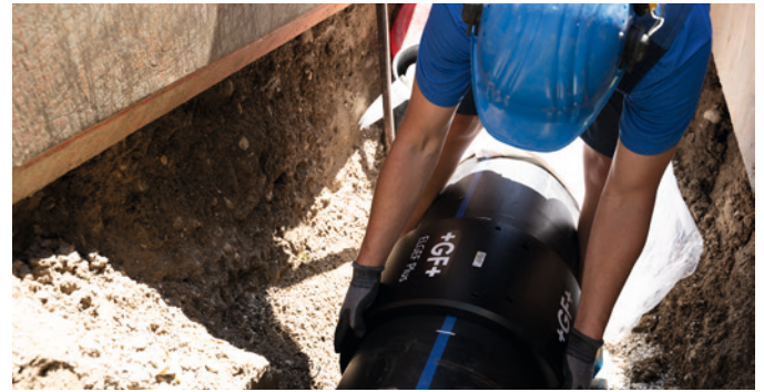
The extra-large inner diameter of the coupler allows easy assembly.
