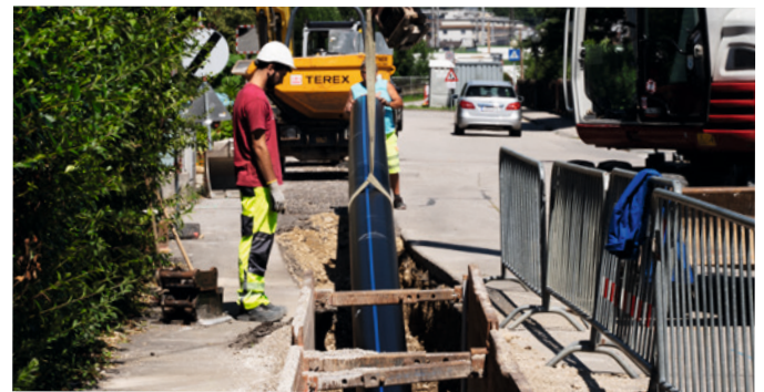
Integrating a 12m long PE pipe in a trench shoring operation.
