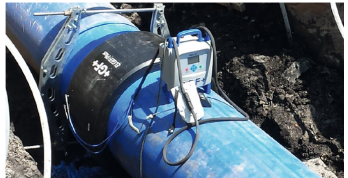
Full product package: ELGEF Plus fittings, rerounding tool and MSA fusion unit.
