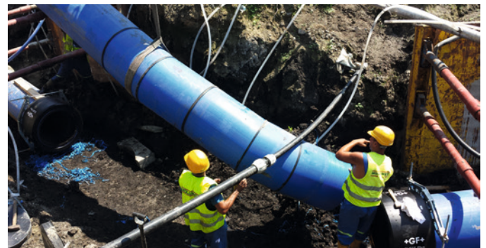
Onsite integration of a segmented bend by easy sliding of ELGEF Plus couplers.
