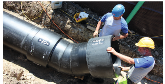
Prefabricated segmental arches were connected using ELGEF Plus couplers, to ensure the system is airtight.
