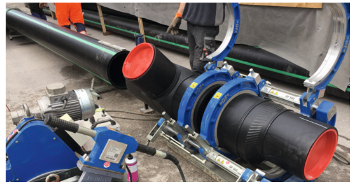
Simple and reliable: butt welding machine GF 500 and GF nozzle fittings.
