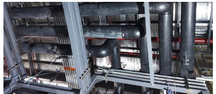
More than 11'000 corrosion-free PE100 fittings help to lower the carbon emissions of NARRA1 by over 135'000kg CO2.
