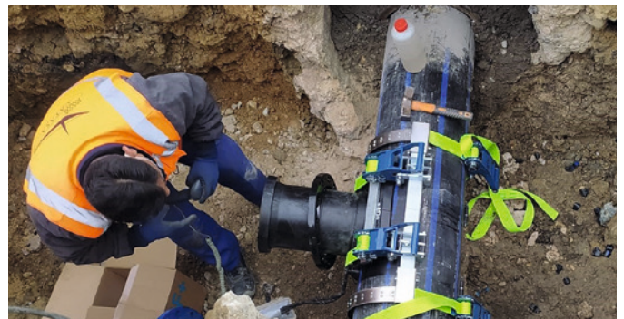
The topload tool supplied by GF Piping Systems allows for a flexible placement of branch saddles without having to cut the pipes.
