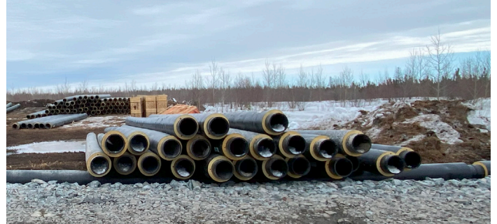
The Tataskweyak Cree Nation enhanced its drinking water system with GF Urecon's solution, installing over 25,000 feet of insulated HDPE pipe to deliver raw water to a new treatment facility.
