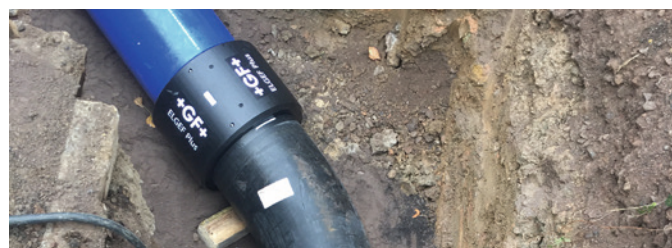
Installation of the new polyethylene firefighting piping.
