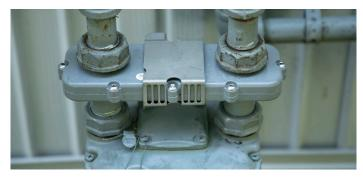
Scheduling and rescheduling to re-light pilots or conduct appliance checks is no longer an issue. The Co-Pilot® Meter Bypass System allows a gas meter to be safely and easily replaced without interrupting service or the need to enter a residence.
