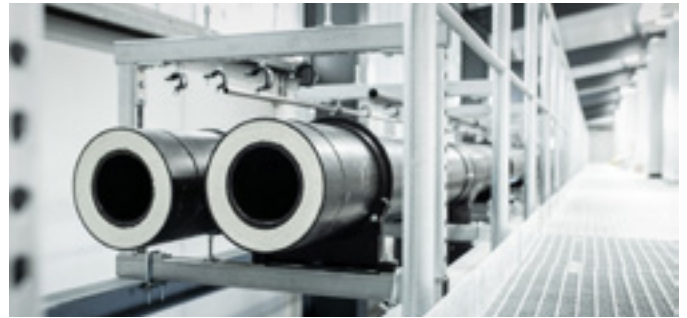
More than 200m of COOL-FIT help Voltavision achieving a climate-neutral cooling system.
