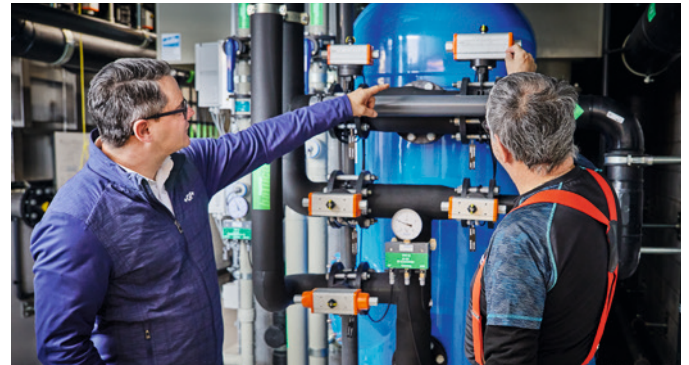
Precise flow rate adjustment for swimming pools with the plastic Butterfly Valve 565.
