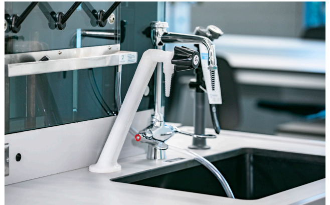
GF AquaTap™ recirculating laboratory faucets installed in combination with In-line flow diverter (IFD) eliminate dead-legs at all points of use to maintain purity throughout the DI water.
