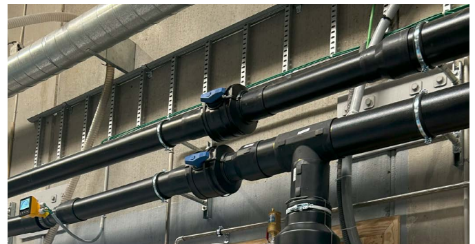
COOL-FIT 2.0 installation performed at heights up to 7 meters. As COOL-FIT is lightweight, installation can be done by one person. A d110 COOL-FIT pipe weighs 5.6 kg per meter. In comparison, an equivalent steel pipe weighs approximately 14 kg per meter.
