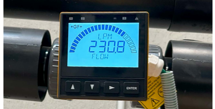
The COOL-FIT 2.0 installation can be upgraded with a 9900 transmitter with a paddlewheel sensor mounted at a height of 3 meters. Yet the flow can easily be read while standing on the floor.
