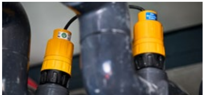
GF measurement solutions offer state-of-the-art solutions for pH measurement and a long lifetime even in harsh environments.
