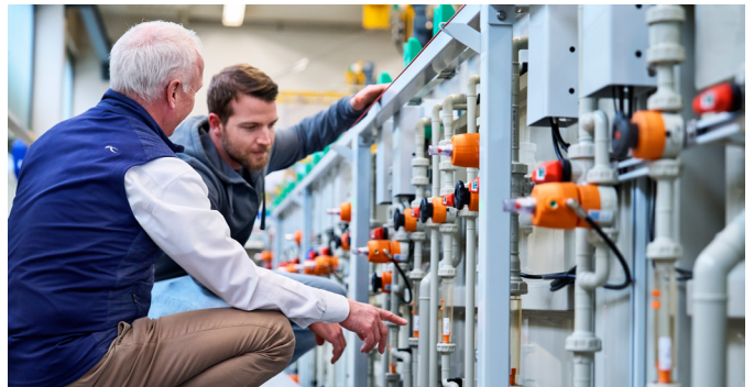
Plating lines require safe, reliable, and automated flow solutions to ensure the highest quality.
