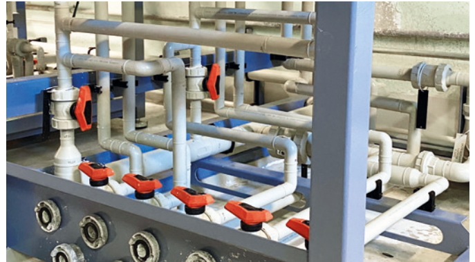
Infrared welded PP-H piping system with 546 Pro ball valves in the foreground.
