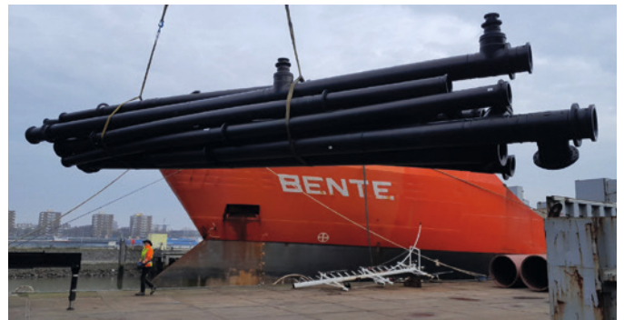
In order to speed up the installation, many pipe sections were prefabricated and custom-made to meet the needs of the customer.
