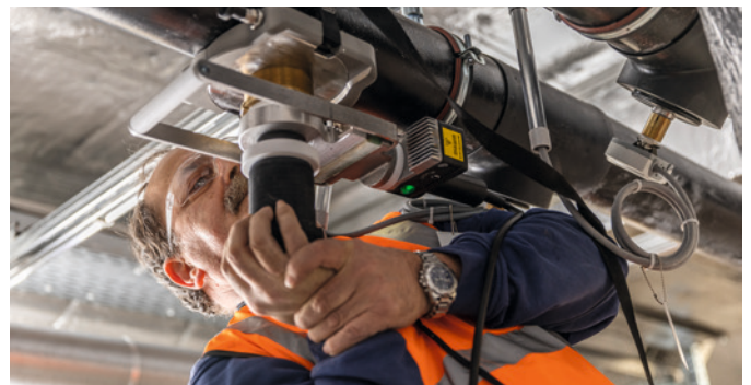
Thanks to the easy and quick installation, the Weld-in port was seamlessly integrated into the existing pipe.
