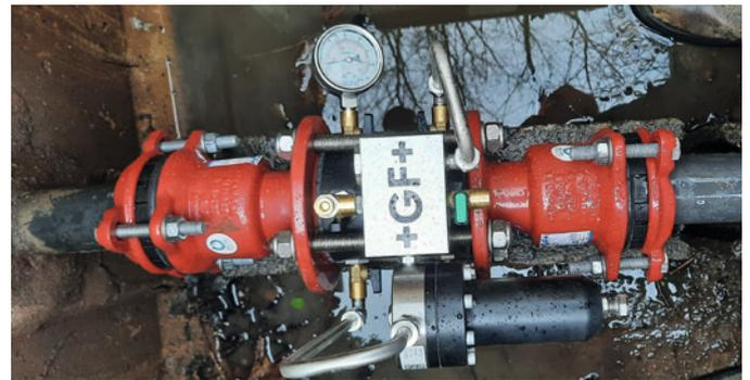
Thanks to its axial flow construction, NeoFlow ensures a stable flow from 1% to 100% opening, even at a small operating differential.
