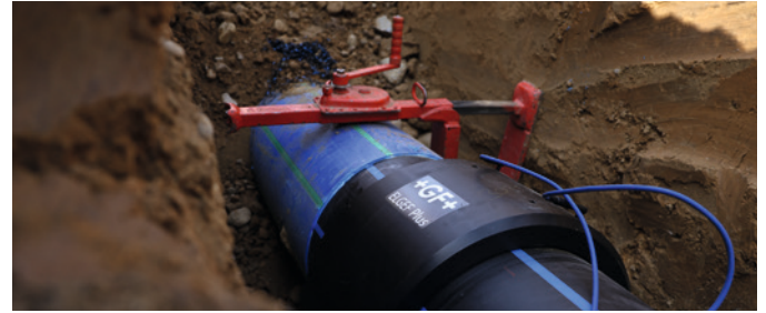
Easy installation of the large-diameter ELGEF Plus Coupler in a narrow trench.
