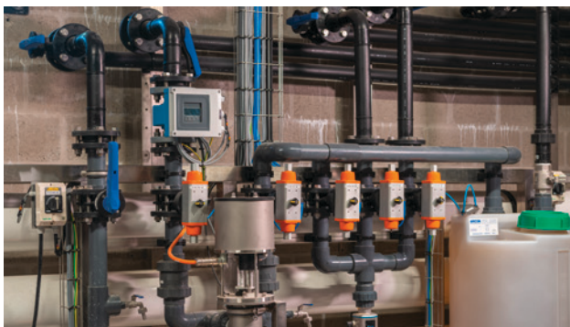
Butterfly valves equipped with pneumatic or electric actuators are used as process and control valves.
