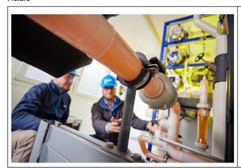
SYGEF ECTFE is an infrared welded plastic piping system that ensures maximum operational stability, and has been designed with a focus on human and environmental safety.
