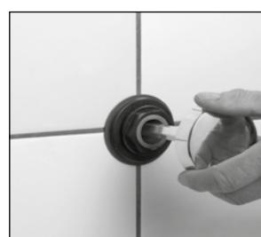
Insert the trimmed valve rod extension into the hexagon of the handle rosette. Insert the rosette together with the actuator extension into the sheath tube and put it over the hexagon of the top section of the valve until it clips on the blind flange.
