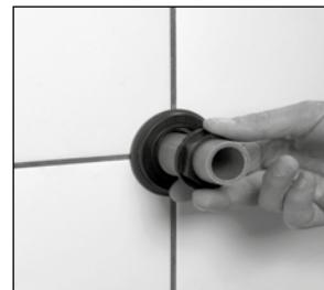
Attach the red or the blue ring (utility markers) to the blind flange and mount it to the sheath tube. Put the coupling nut on the tube end and screw it two turns by hand.
