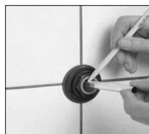
Insert the hexagonal valve rod extension into the sheath tube all the way to the stop. Mark the extension to be flush with the leading edge of the coupling nut, trim it at right angles, and bur it.
