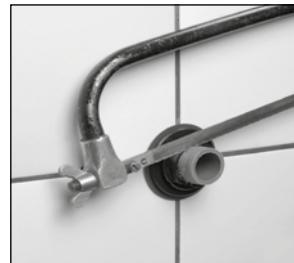
Trim the sheath tube to be flush with the leading edge of the nut.
