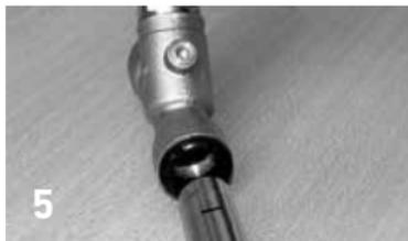
Control optically the body for cleanliness before putting in the pipe and correct seat of the O-ring. By easy turning push in the pipe, until it reaches the marking.
