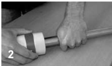
Deburr smoothly the pipe internally and externally with a commercial deburring tool.
