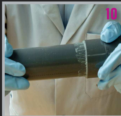
Connect pipes and fittings to its full depth without twisting
