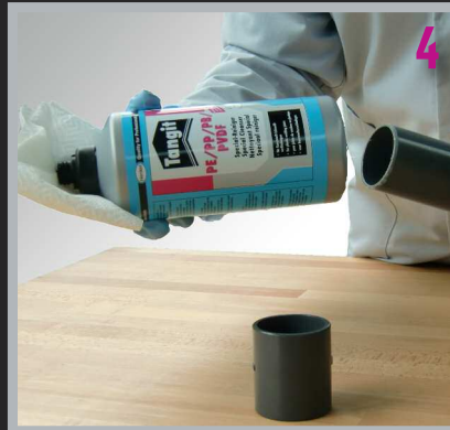
Cleaning of pipe and fitting
