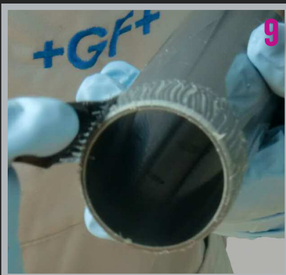
Dispense adhesive on pipe with plastic brush
