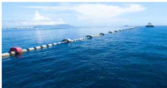
The tugboat tows the piping system prior to its submersion.
