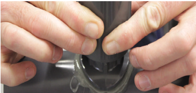
Firmly press the saddle onto the pipe
