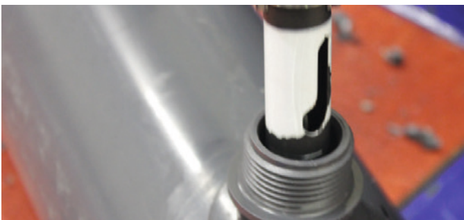
Apply solvent cement to the pipe
