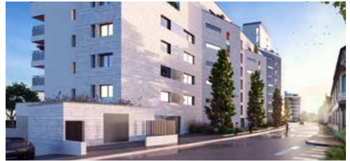
The drinking water installations for the high-quality apartments meet the highest hygiene standards. (Visualizations: AEA Architects).
