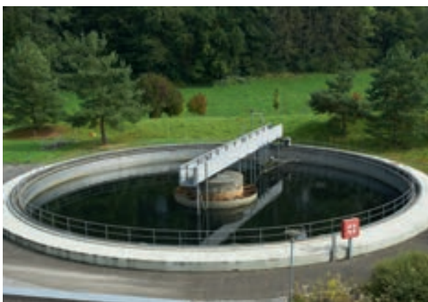
Wastewater treatment plant, ARA Bülach, Switzerland.
