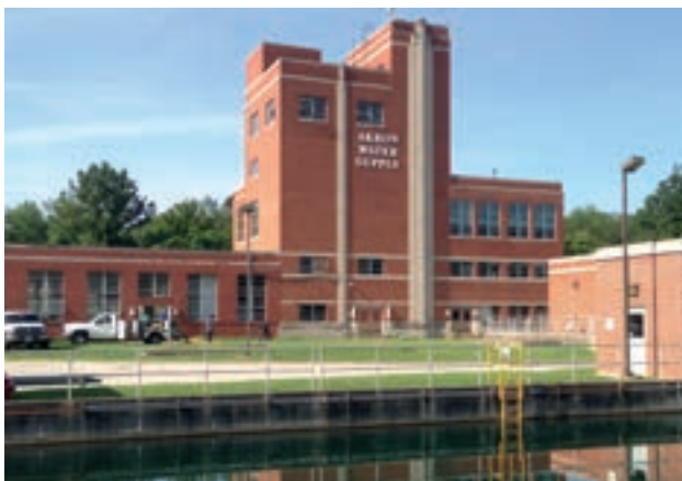
Potable water plant, City of Akron, Ohio USA.
