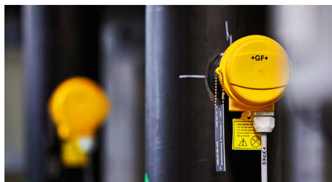
Magnetic-inductive flow meters monitor reliable operation.
