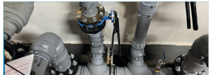
Hot water manifold after replacement.
