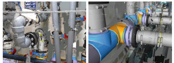
3D Scanning by MecShip to design the replacement of the hot and cold water manifolds (provided by MecShip/CCL).
