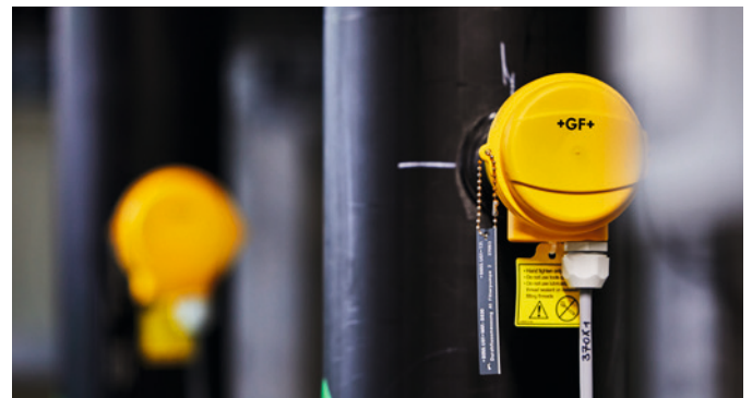
Magnetic-inductive flow meters monitor reliable operation.
