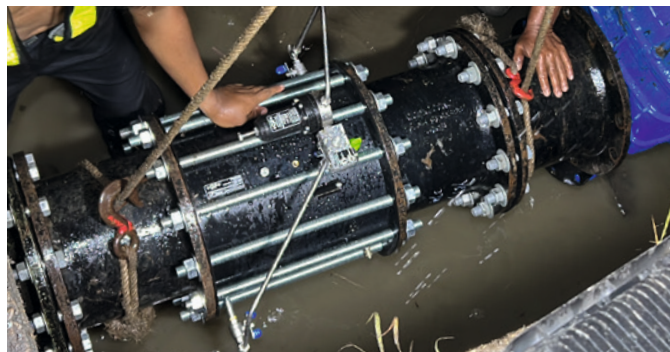
The installation took place without any complications.
