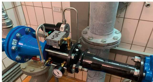
Faster and easier installation thanks to the light NeoFlow polymer pressure regulating valve and wafer-type arrangement.
