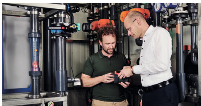
Pieter Loose, CEO of Ekopak and Bart Van Bastelaere from GF Piping Systems in front of an Ekopak container.
