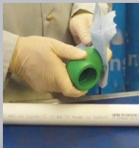
Clean the fitting
