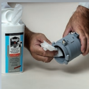
Clean pipe and fitting
