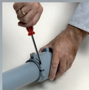
Insert pipe into fitting and tighten screws
