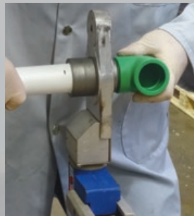
Heat up pipe and fitting
