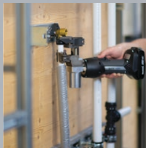
Engage pipe to the fitting inside the tool jaws. Press the tool trigger to simply complete the jointing process.
