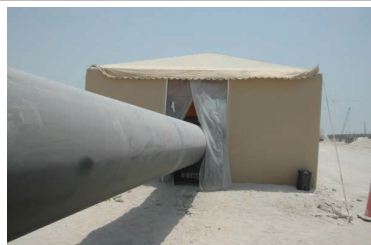
Protecting the welding zone using a tent
