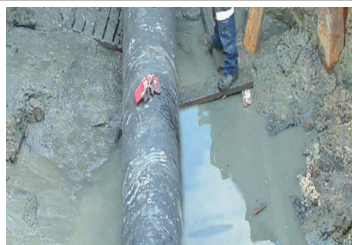
Water residues must be pumped off
