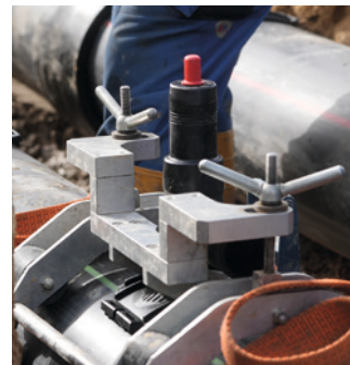
Among the components being used for the sustainability project are pressure tapping valves from GF Piping Systems. These valves can be rotated through 360° prior to welding.
