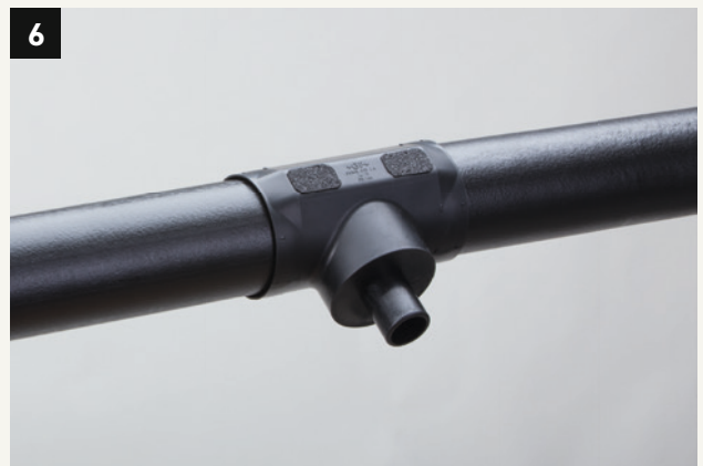
6 Seal the welding connectors with the attached insulation plugs - done!
