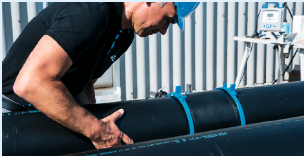
Slide the ends of the pipe into the fitting as far as the marking. Then remove the mounting aid.
