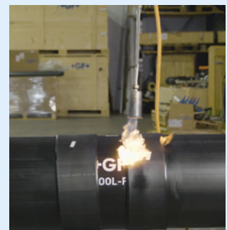
Seal the jointing face between the fitting and pipe with sealing tape and shrink the shrink sleeves.
